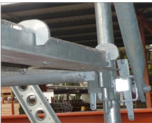
Photograph 6 –Lock hooks over transom.
