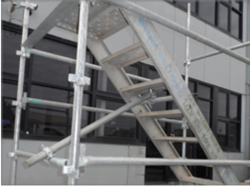
Photograph 8 – Prop underneath stair module.
