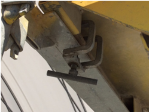
Photograph 10 – Clamp securing stair module to transom.
