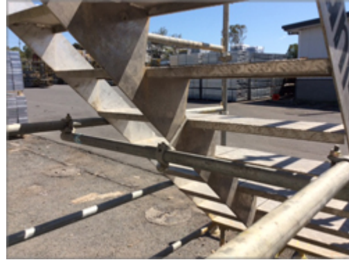
Photograph 9 – Horizontal tube under stretcher stairs.
