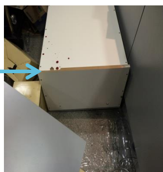
Point where side of carcass failed
