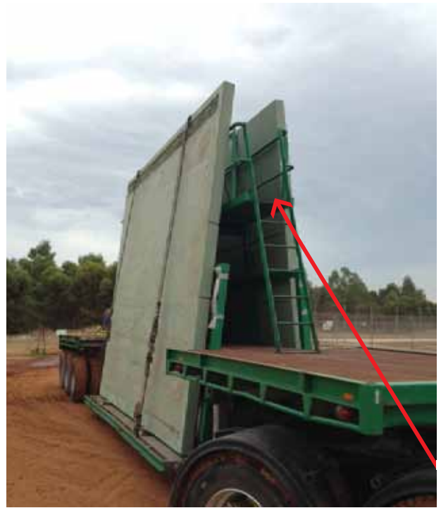
Above: Where reasonably practicable, engineered fall protection and access should be provided.
