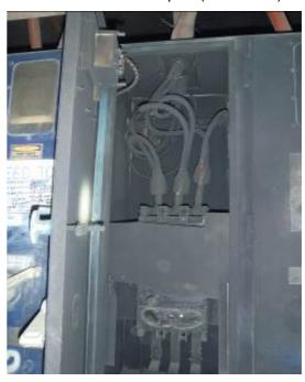
The electrician received serious burns to the upper part of his body and both sides of his face. The electrical fault was cleared by overcurrent protection on the 11kV side of the substation.
