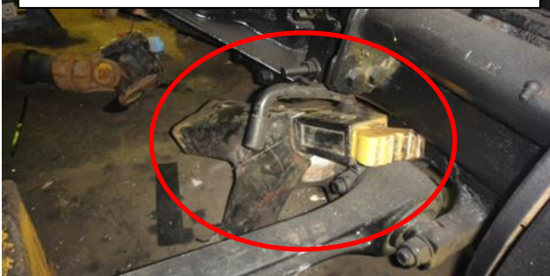
Failed Support Stand under Wheel Pos 3
