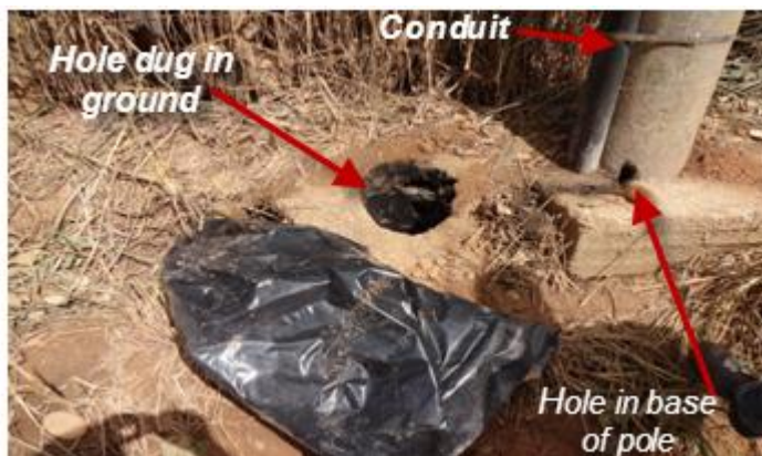
The base of the pole showing the hole they were digging.
